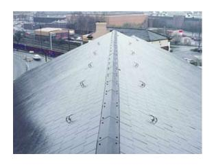
**KEE ROOFPOINT** fall arrest anchor solutions provides a range of permanently fixed roof anchor points designed to promote safer working on roofs. **ROOFANKA**, **RIDGANKA** and **POSTANKA** all offer solutions to solve different access problems when used correctly in conjunction with the appropriate PPE (Personal Protection Equipment).
