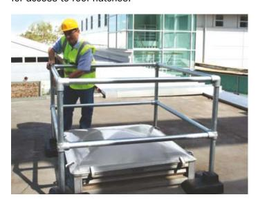
The **KEE DOME** structure is safety compliant, remains completely free-standing and eliminates the risk of damage to the roof membrane.
