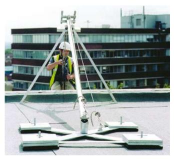
**WIREANKA** is the first anchor device to be approved for use as supports for Class C horizontal flexible safety lines.
