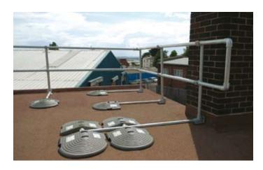
By using a correctly installed and tested **KEEGUARD** roof edge protection system you can ensure the health and safety of anybody who goes onto a flat roof. **KEEGUARD** is a modular free standing system that has been fully tested and approved which does not penetrate the roof membrane.
